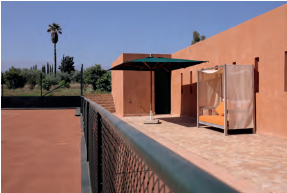
Clay tennis court with club house and shower
